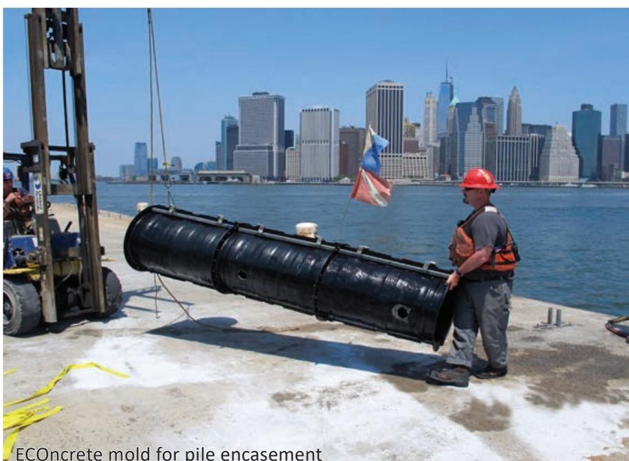
ECOConcrete mold for pile encasement
