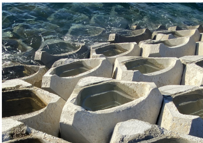
SITE 2: Coastalock units fit together to provide further stabilization of the breakwater and create ecological uplift opportunities through the creation of diverse habitats from inter-tidal to submerged zones depending on the unit orientation.
