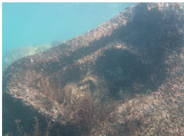
SITE 2: Coastalock units fit together to provide further stabilization of the breakwater and create ecological uplift opportunities through the creation of diverse habitats from inter-tidal to submerged zones depending on the unit orientation.
