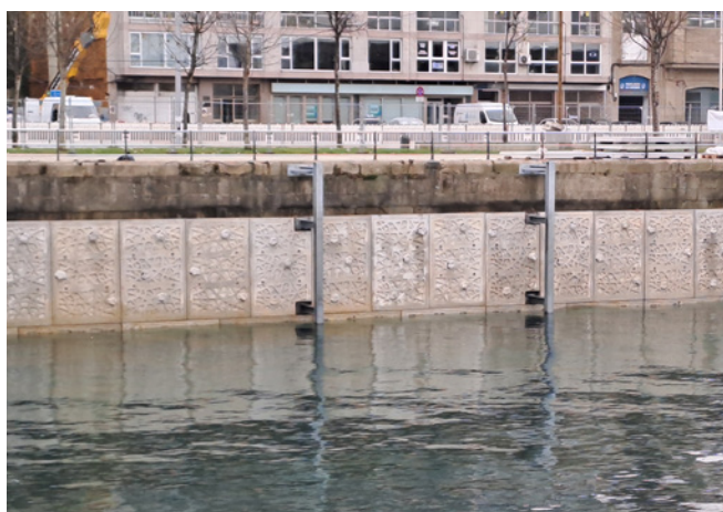
SITE 1: Installation of ECONcrete eco-engineered seawall panels on the A Laxe dock, adjacent to the 'Nautilus' observation deck.
