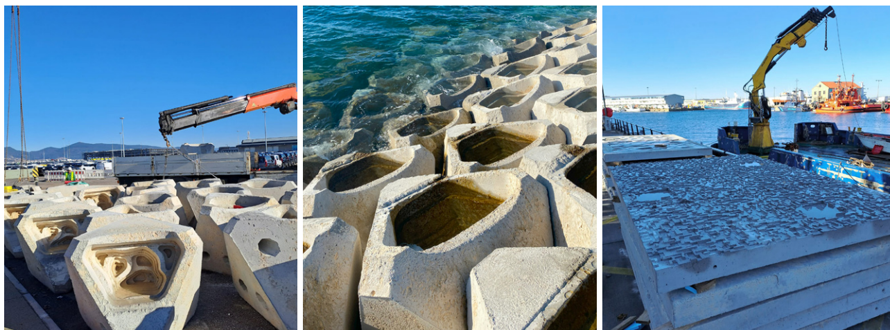
Figure 2. Left: Coastallock units manufactured with bio-enhancing Admixture by a local precaster lining up for installation. Middle: Coastallocks shortly after installation in the Bouzas revetment. Right: EConcrete’s nature-inclusive Azouri Seawall design is proven to create diverse habitats for shelter, attachment, and growth, and to maximize surface area.
